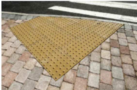
3- Proposed blister paving flags to pedestrian crossings
