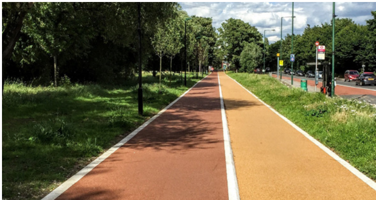
9- Proposed coloured bitmac to cycle route to engineer's spec.
