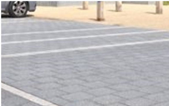
5- Proposed permeable paving to car parking spaces to eng. specification
