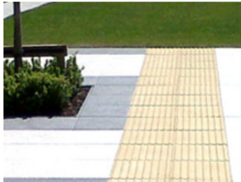
6- Proposed courduroy hazard warning paving flags to pedestrian crossovers
